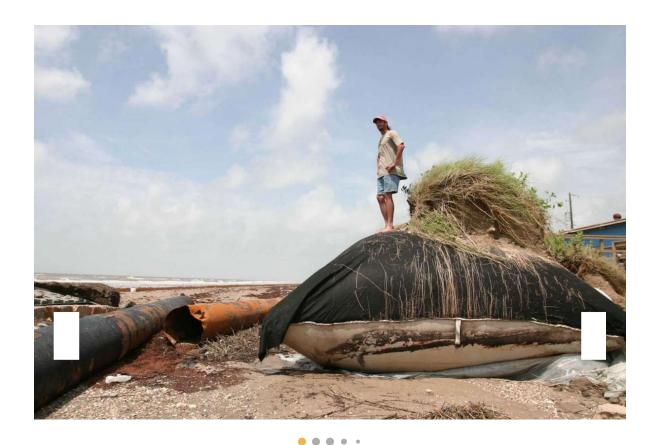
File photo shows Chuck Hale surveying the damage to a geotube, a sand-filled tube, that was exposed at Rollover Pass near Gilchrist on the Bolivar Peninsula on July 16, 2003. Residents said the protective tubes were covered with three feet of sand until Hurricane Claudette battered the Texas coast.
